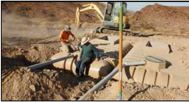
Prepping for and placing the tanks
