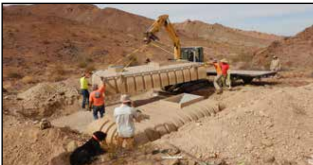
Prepping for and placing the tanks
