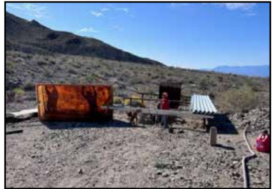
Tank and metal removed by SGQF/SCBS volunteers
